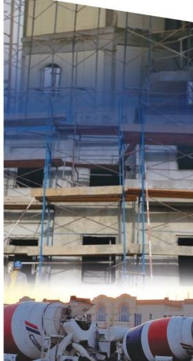
CEMEX Shotcrete concrete is a specially designed concrete developed for use with compressed air spraying equipment. Shotcrete is a fast and effective way to apply a concrete in areas where using conventional concrete would be difficult. CEMEX Shotcrete also forms an integral part of an innovative low cost, low carbon housing solution
